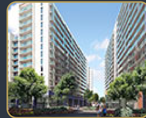
Chapel Wharf, M3 Dandara Living
